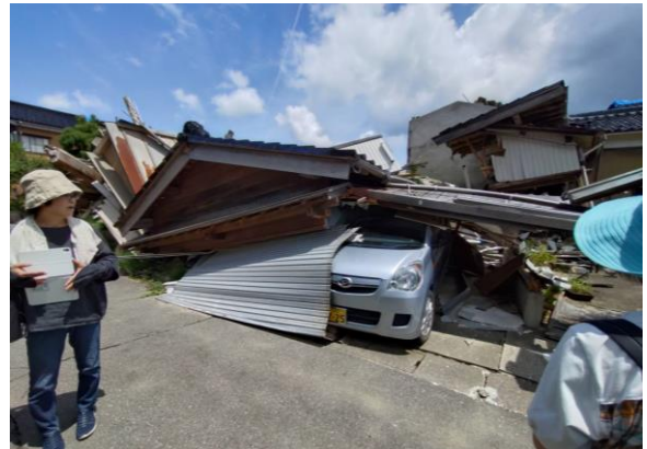
Suzu city, Ishikawa Prefecture, one of the areas hardest hit by the New Year's Day earthquake. Demolition work has fallen far behind the schedule, hampering the recovery efforts (July 19)
